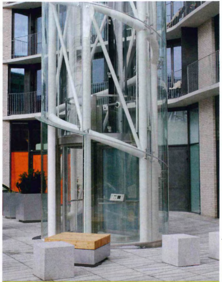
The Icon Tower is an 84-m-tall glass observation tower erected in Oslo, Norway. The elevator includes a custom all-glass cabin (which becomes transparent when above neighboring buildings) with a glazed floor and ceiling.
