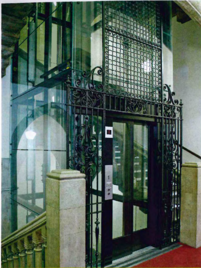
The Royal Courts of Justice were opened in London in 1882 by Queen Victoria. In 2009, the so-called "Black Lift," a nine-person elevator, was removed and replaced with a 13-person elevator installed within a steel and glazed-glass structure. For this modernization project, automatic Sematic 2000 B framed glass lift doors with special-depth kickplates were chosen.
