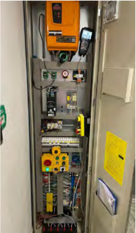
An example of a complete Wittur Electrical Modernisation package, with door operator, gearless drive and inverter.
