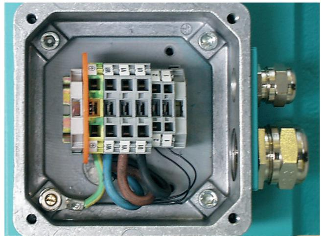
Terminal box for motor connection
