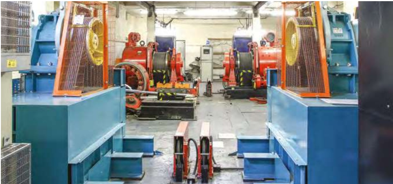
The latest-generation gearless drives from Wittur are more energy-efficient and take up much less space than older-generation ones (which can be seen in the background of this machine room during its modernization project).
